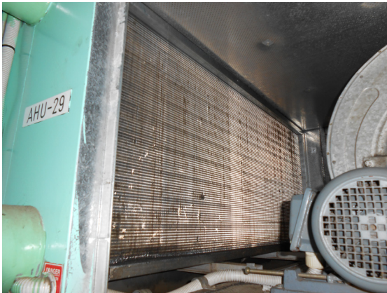
HVAC Air Handling Unit before UVC installation Photo: Beyond Energy Solutions
