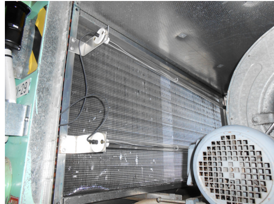
HVAC Air Handling Unit after UVC installation Photo: Beyond Energy Solutions
